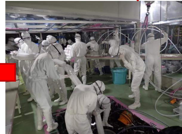
Mini-balloon installation into KamLAND
