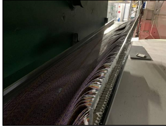
ADC cables: to patch panels↑; to DAQ rack↓
